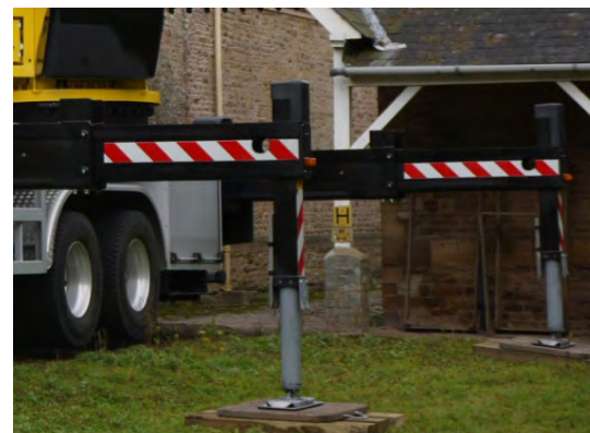
MEWP Outriggers on Pads and Timbers
