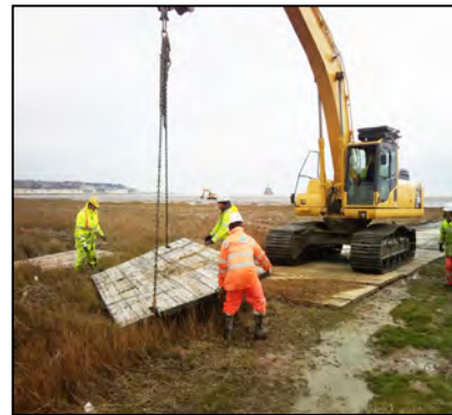
Positioning of Timber Mats
